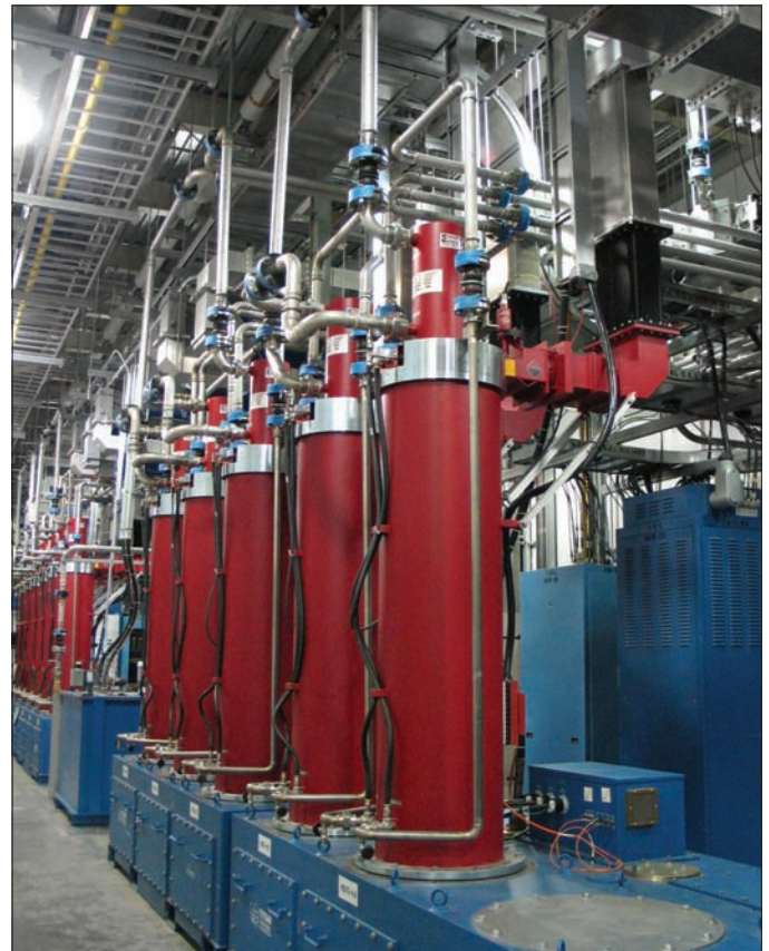
The conference included a tour of the Spallation Neutron Source, with its impressive klystrons. (Courtesy Pamela J Kite ORNL/NScD/RAD.)
