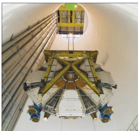
The small wheel made the 100 m journey into the underground ATLAS experimental cavern, landing safely at the bottom in an hour and a half.
